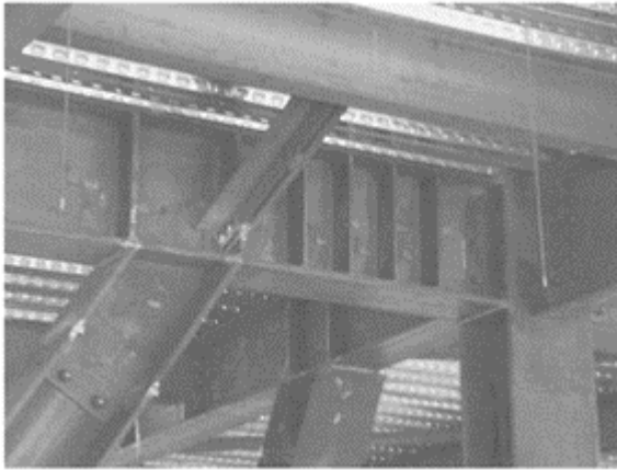
FIGURE 16.6 Typical link detail (courtesy of Structural Engineers, Inc.).
