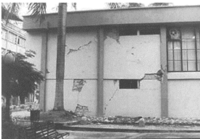
FIGURE 17.14 Damage to unreinforced masonry
