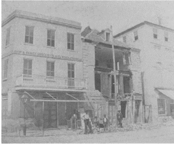
FIGURE 17.3 Damage to masonry in the Charleston, SC, earthquake of August 31, 1886.
