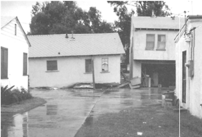
FIGURE 18.6 Partial collapse of split-level home in the 1971 San Fernando earthquake. (Source: National Information Service for Earthquake Engineering (NISEE) and University of California Earthquake
