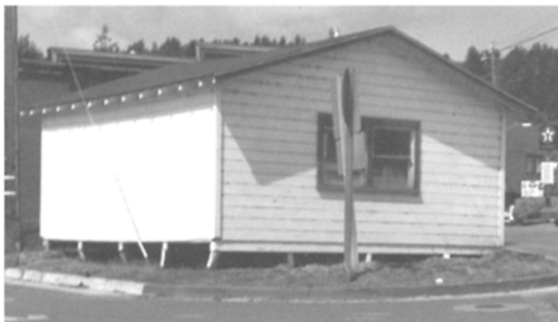
FIGURE 18.10 Racked post and beam supports on house without cripple wall sheathing in the 1992 Cape Mendocino earthquake.
