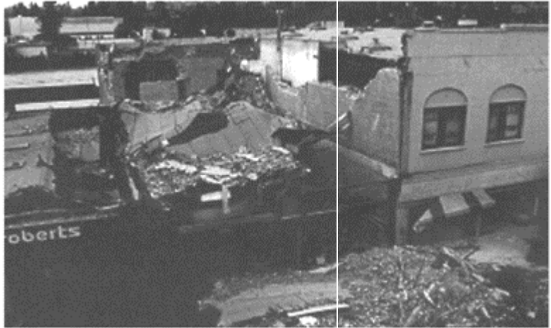
FIGURE 17.7 Collapsed unreinforced masonry buildings in Santa Cruz after the Loma Prieta earthquake. (Photo by the International Masonry Institute.)
