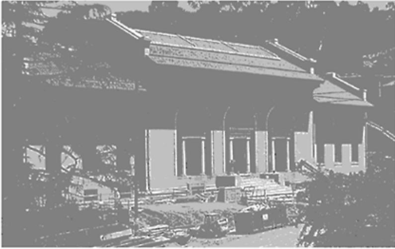
FIGURE 11.5 Hearst Memorial Mining Building on the University of California, Berkeley Campus. An example of base isolation retrofit.
