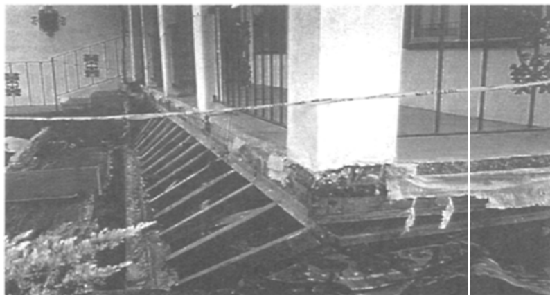
FIGURE 18.11 Single-family residence with collapsed cripple walls in the 1994 Northridge
